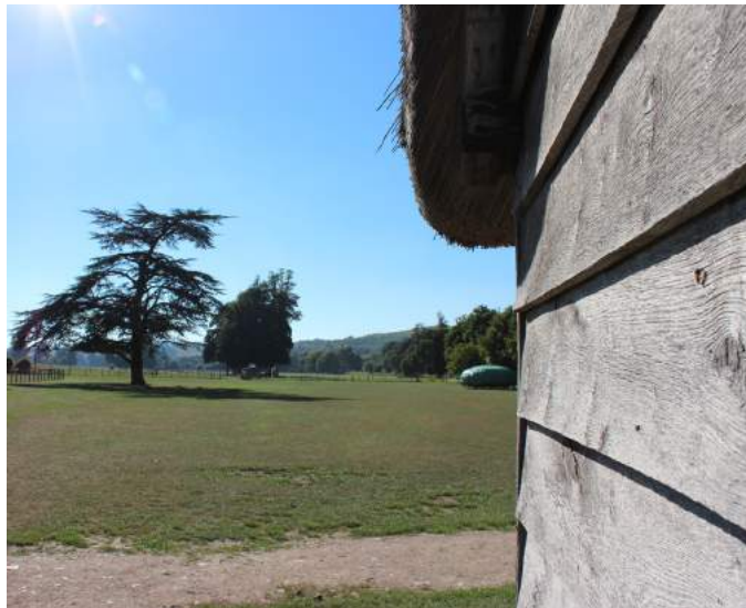
Traditional timber boarding
