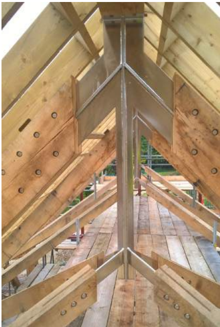
Slotted Structural Junction
