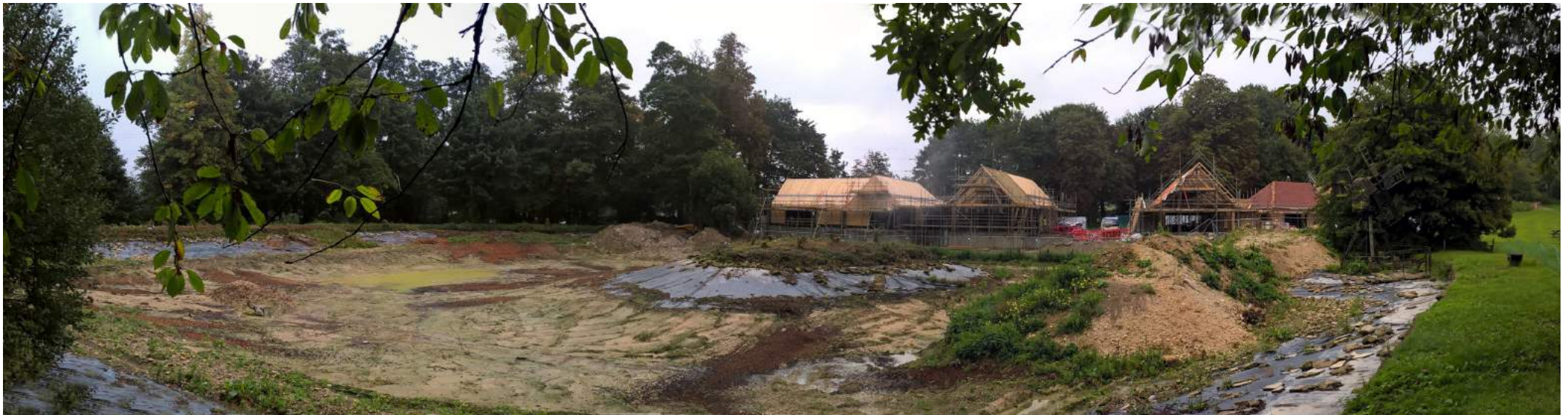
Existing & Mid-Construction View looking East over Millpond
