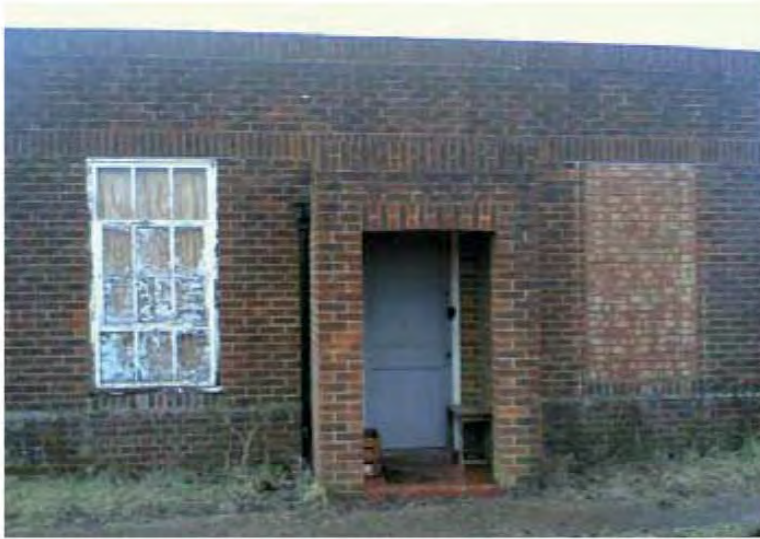
fig 3.4 Existing pump house
