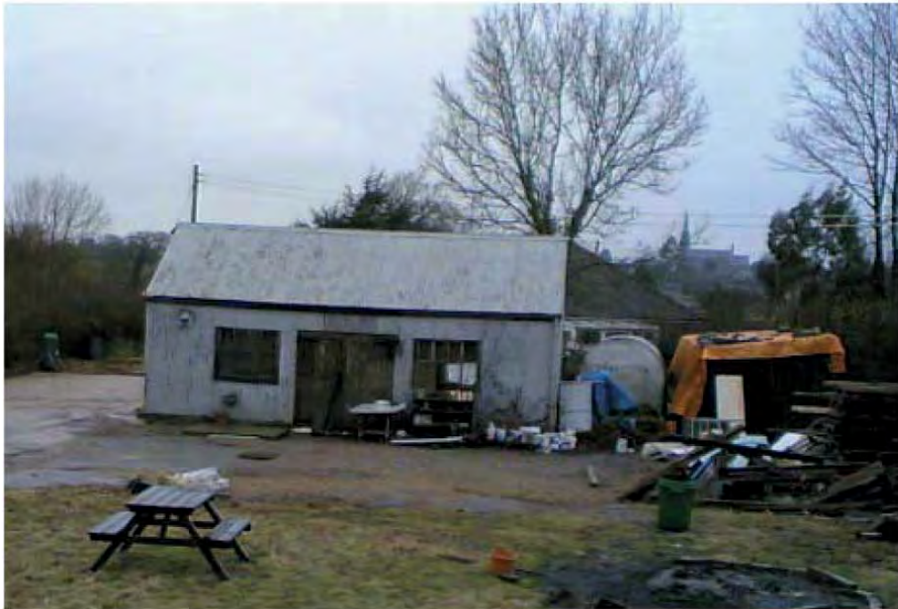
fig 3.5 Existing dilapidated tin shed
